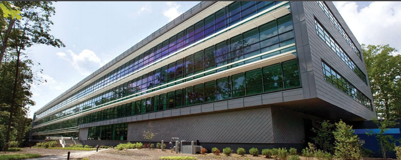
Photo: CarMax office location in West Creek Business Park
