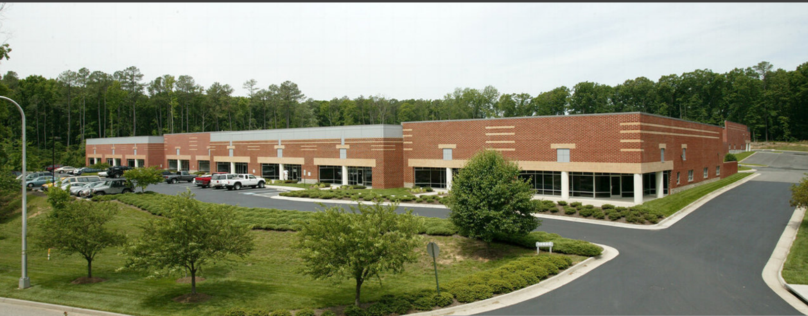
Photo: Manakin Trade Center existing industrial space
