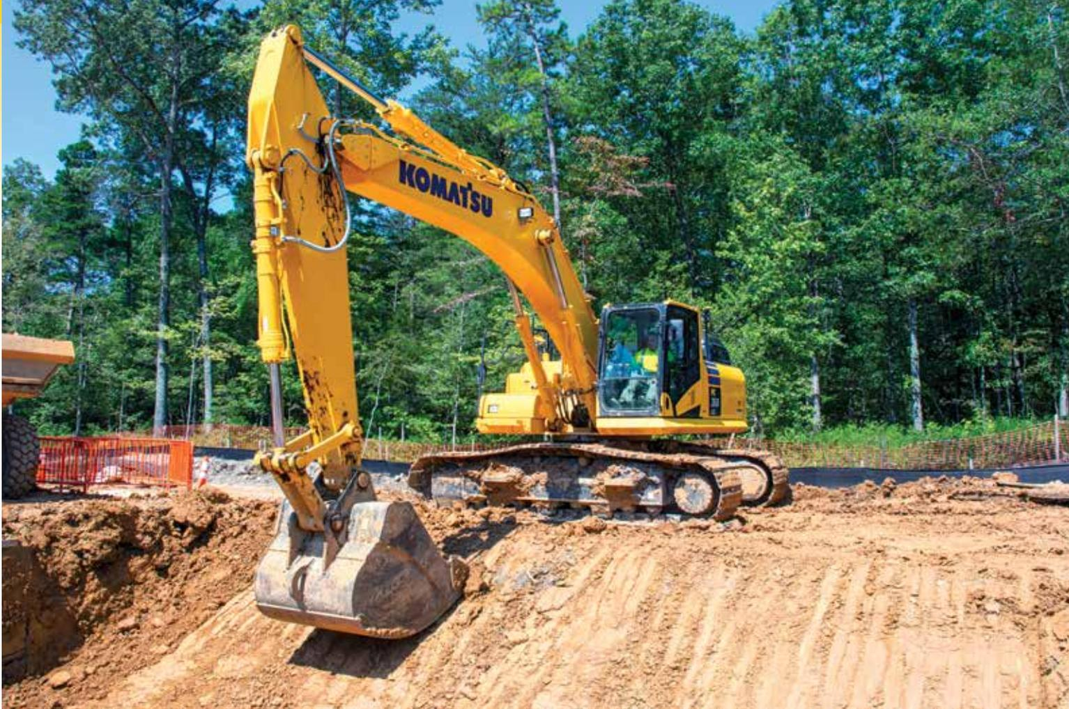
Komatsu *intelligent* Machine Control excavators, including this PC360LCi-11, are go-to machines for Liesfeld Contractor, which puts them to work excavating, digging trenches and constructing ponds. “They have the versatility to move mass quantities of materials as well as do precision work such as slopes, so we were able to construct a relatively large pond rather quickly,” said Technology/GPS Manager Chris Ashby.
